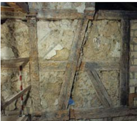
Fig. 9. View of the western wall of the hallway on the second residential floor. Remnants of paint and the closed-off recess for the top step point to the original location of the stairs.
