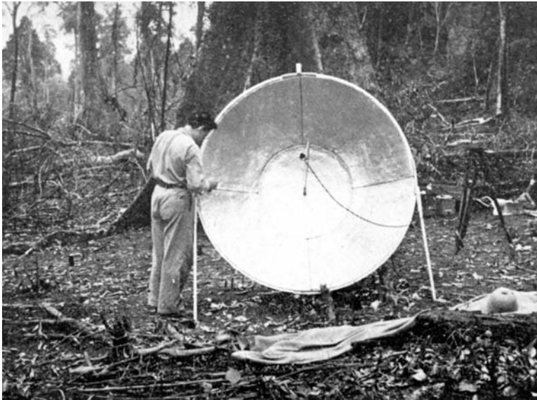
Fig. 16.1 Clarence R. Carpenter and his parabolic reflector microphone in Chiang Dao, Chiang Mai, Thailand, 1937. This installation was used to record the calls of wild gibbons on disk. Photo from Carpenter (1940, p. 26; Johns Hopkins Press, Baltimore)
