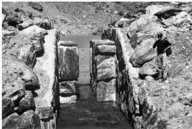
Fig. 14. New (lowered) flood-release (overflow) structure with regulating gates at proglacial Lake No. 1 (photo W. Haerberli, July 2000).
