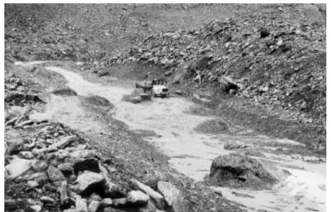
Fig. 13. Excavation of a drainage channel for ice-marginal Lake No. 3 (photo A. Kääb, 1995).
